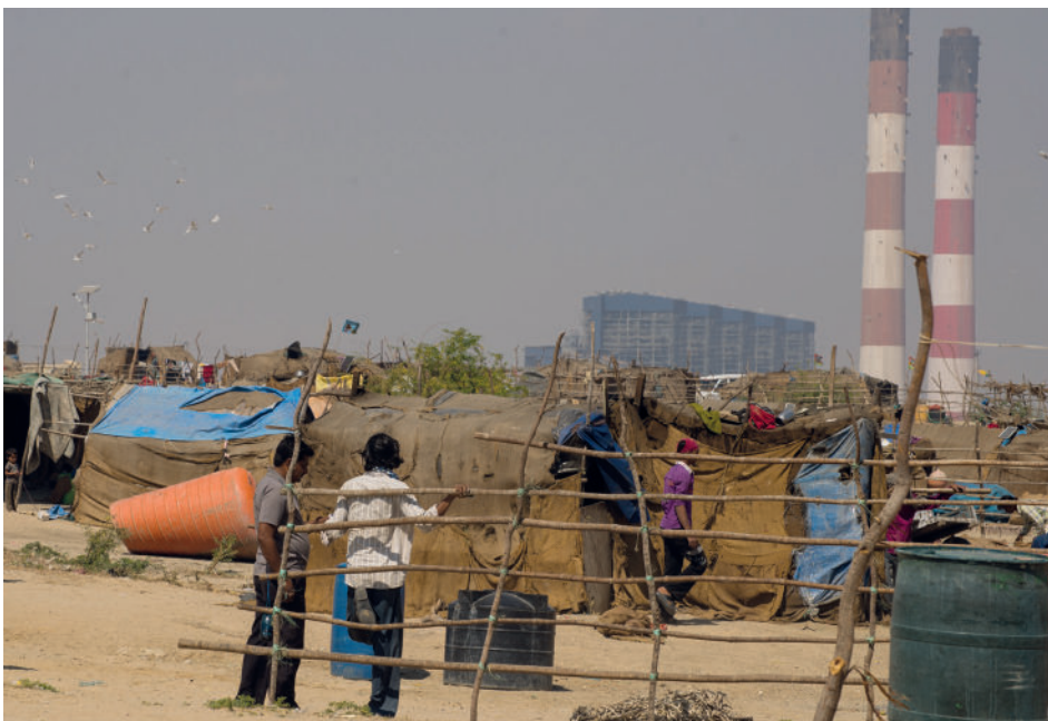
Settlement overlooking the Tata Mundra coal power plant
