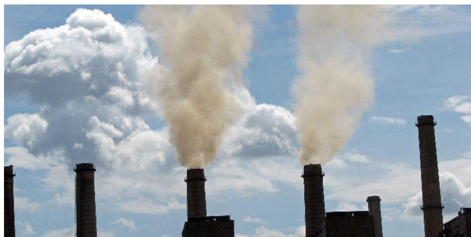
A coal-fired power plant in Kosovo.
